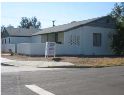
Where the sidewalk ends (install sidewalks where there are gaps)
