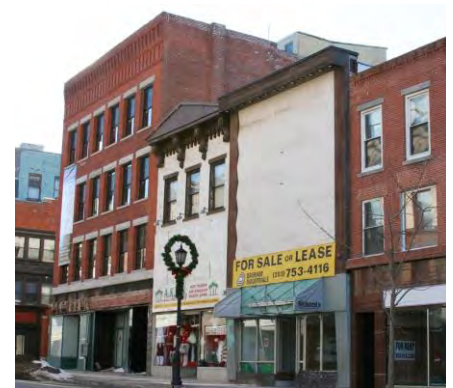
Before façade improvements
